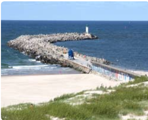
The Waterbreak at Liepāja
