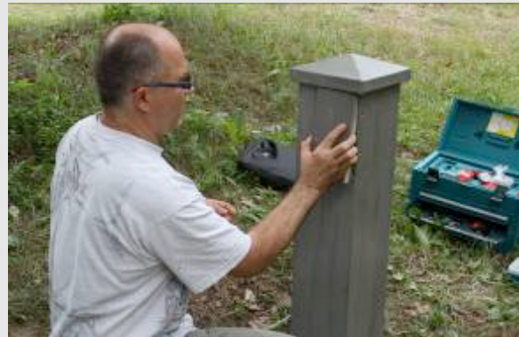
Fig. 29. Electronic counter is hidden in the imitation of barrier post
