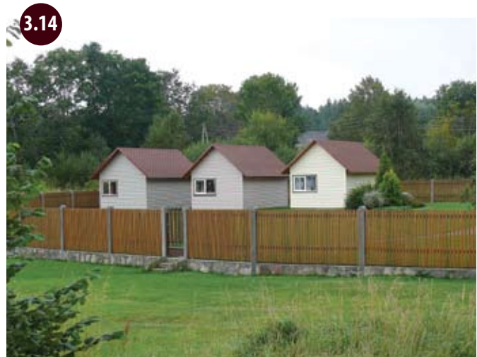
Fig. 3.14 – Not advisable usage of colours, as well as the layout of the construction volume, their proportions and the fence solutions that are not characteristic of coastal construction.
