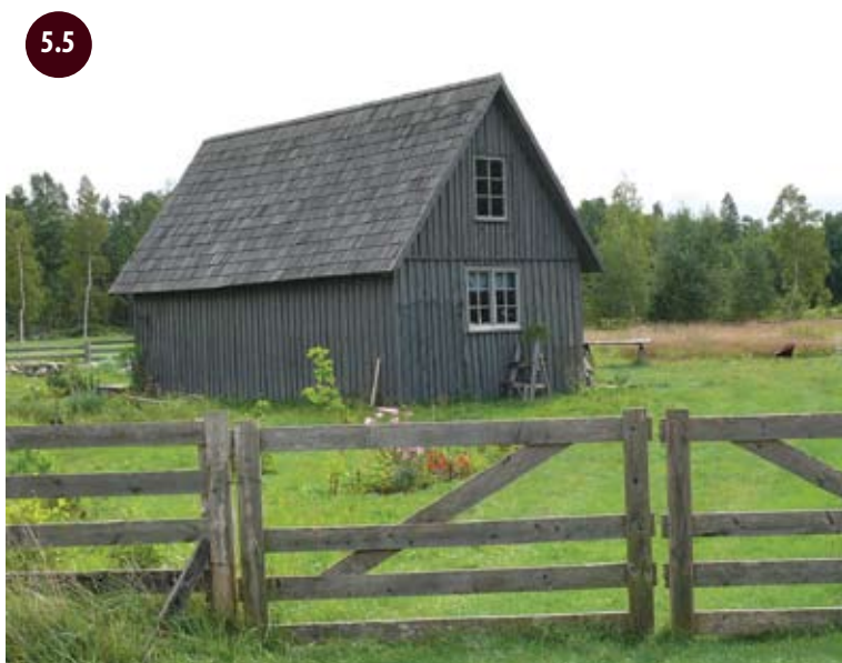
Fig.5.5. An example of inconspicuous transformation of a former household building into a dwelling house. The vertical board upholstery characteristic of household buildings is maintained.
