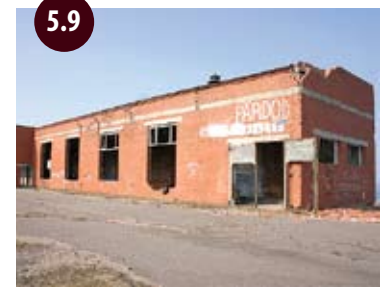
The wreck of the pumping station prior to the reconstruction (Fig.5.9) and the dwelling house afterwards (Fig.5.10).
