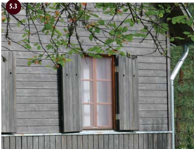
Fig.5.3. A good tonal solution. The practicality in detail solutions characteristic of the coastal construction has been observed in the reconstruction of a dwelling house.
